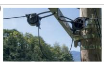
Once the cable is tensioned, tighten the integrated cable tie.
