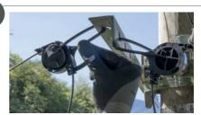
Bring the cable out from the bottom part of the clamp by placing it behind the retaining tab. Lock the bail onto the body.
